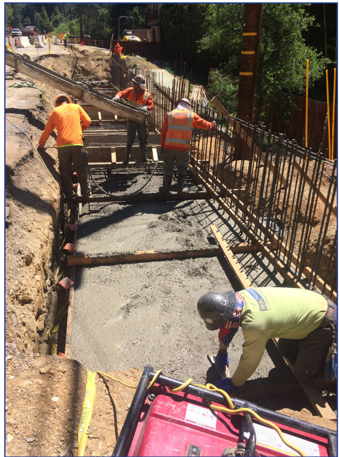
Pouring Retaining Wall Footing
